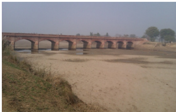
Fig. 4. Side Embayment and Widened section at 97.61 km of UJC
