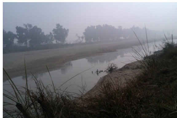
Fig. 3. Inadequate freeboard at 97.61 km of UJC
