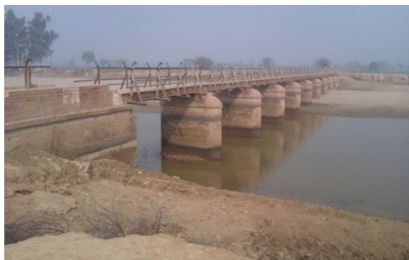
Fig. 5. Damaged Deck Slab and parapet of bridge at 122.6 km of UJC
